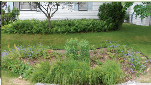
City of St. Cloud rain garden one year after planting
