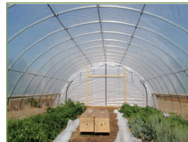
Seasonal High Tunnel constructed in 2010 and 2011. 2178 sq ft each
