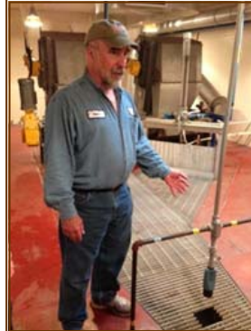
Figure 2 Community Leader Kevin Beadles hosted a tour of the Elk River Waste Water Treatment Facility
