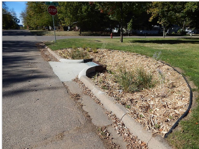
Figure 1: Sherburne County curb-cut rain garden
