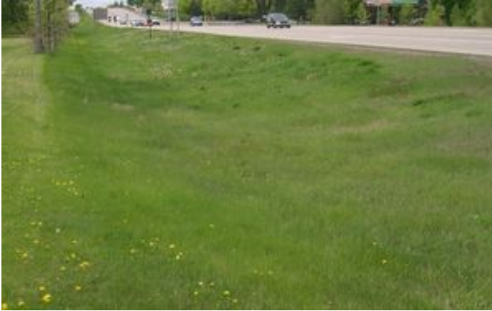
Figure 2: Vegetated swale. Photo by MN Pollution Control Agency (MN Stormwater Manual).
