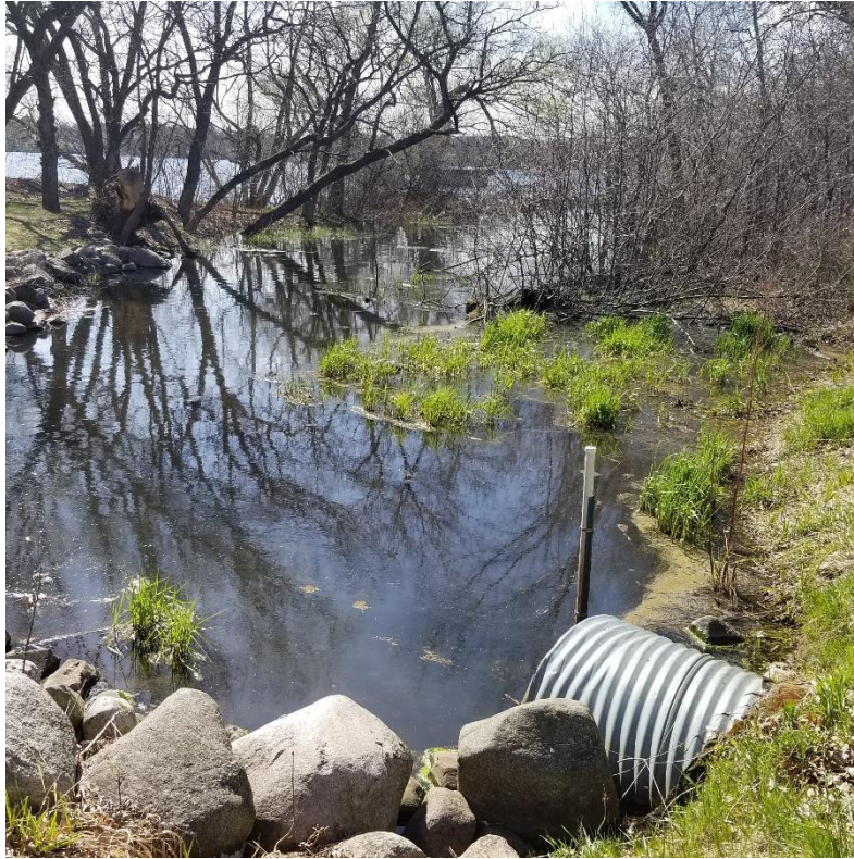
Figure 17. Station 100 Looking downstream.
