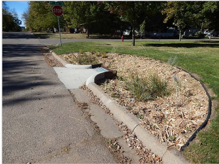
Figure 4: Sherburne county curb-cut rain garden. Photo by Sherburne SWCD.
