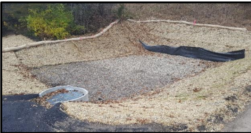
Above: A slotted drain intercepts stormwater several feet before it reaches the lake at the public access location. Infiltration through sandy soils will treat the stormwater before releasing it to the groundwater table.
