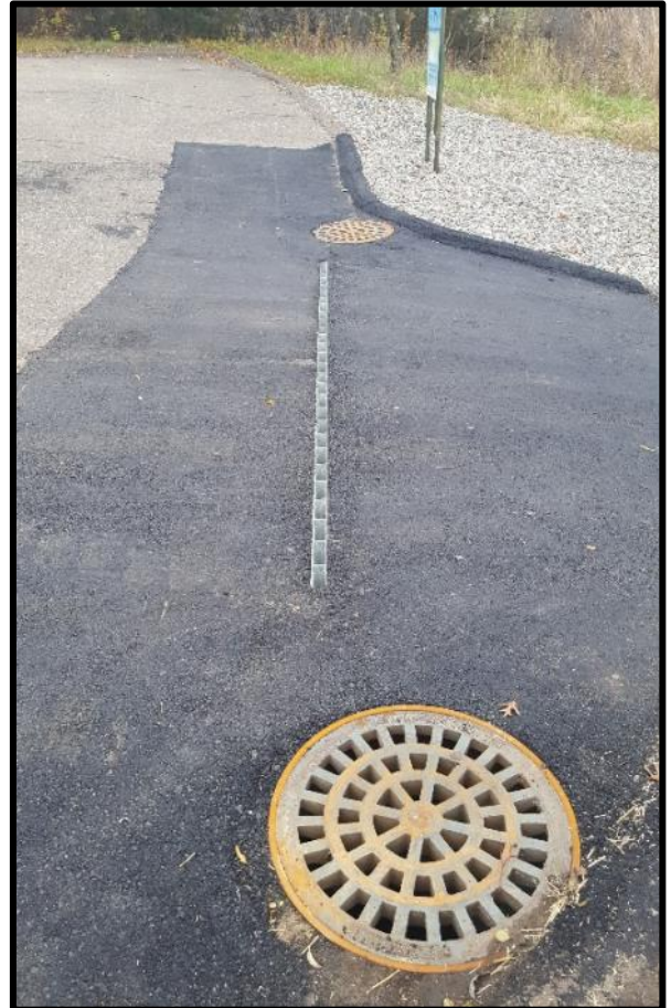
Above: A slotted drain intercepts stormwater several feet before it reaches the lake at the public access location. Infiltration through sandy soils will treat the stormwater before releasing it to the groundwater table.
