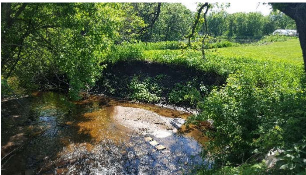
Figure 8 (above left). PMA 2 stormwater pond inlet. PMA 2 drains to this pond and in 2016 a high degree of erosion was noted.
