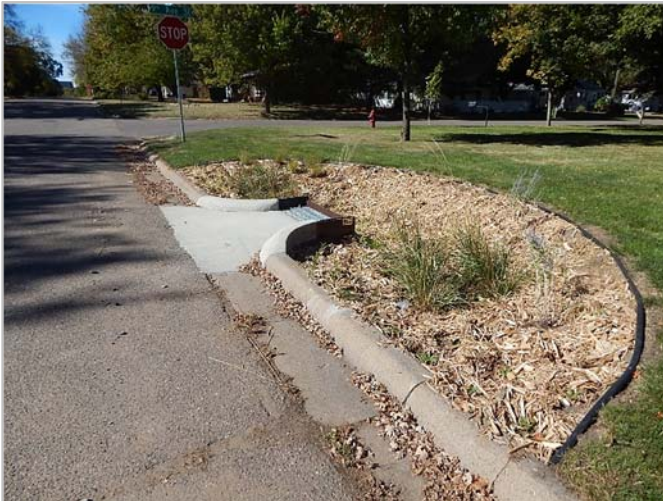
Figure 4: Sherburne county curb-cut rain garden.
