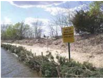
Shoreland buffer in progress at the point on Big Lake. Bundles of pine trees thinned from a Christmas tree farm will protect the new plants from waves. (Submitted photo.)
